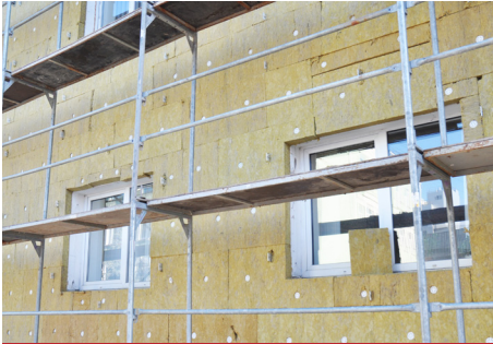
EXTERNAL WALL INSULATION
